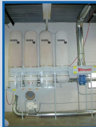
Dustek A/PS-3 connected to a Dustek W1500 4-bag 15HP Collector
